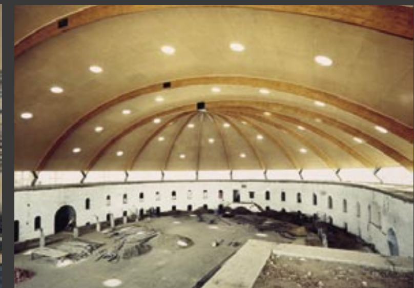
Interior of sport and culture center the Arena in Deurne, erected in 1959-1960 with beams by De Coene after a design by architect Renaat Braem
