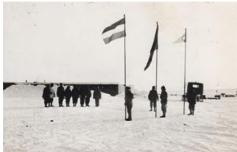
The Belgian-Dutch expedition to the South Pole (1964-1977) in front of the research station, built with prefab elements by De Coene ARCHIVE STICHTING DE COENE VZW
