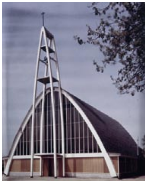
Facade of the Sint-Laurentiuskerk in Lokeren after designs by architect Jan Windels; the bell tower was also executed in laminated wood. First prize, Belgian National Architecture Contest, 1955 ARCHIVE STICHTING DE COENE VZW
